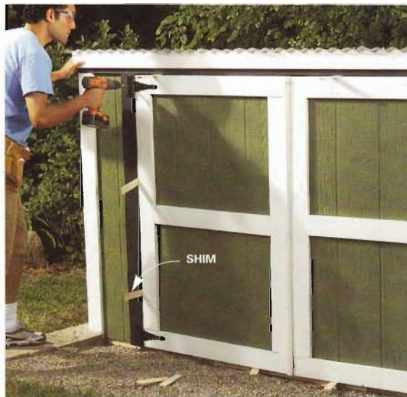
9 Hold the doors in perfect position with shims. Then screw on the hinges.
