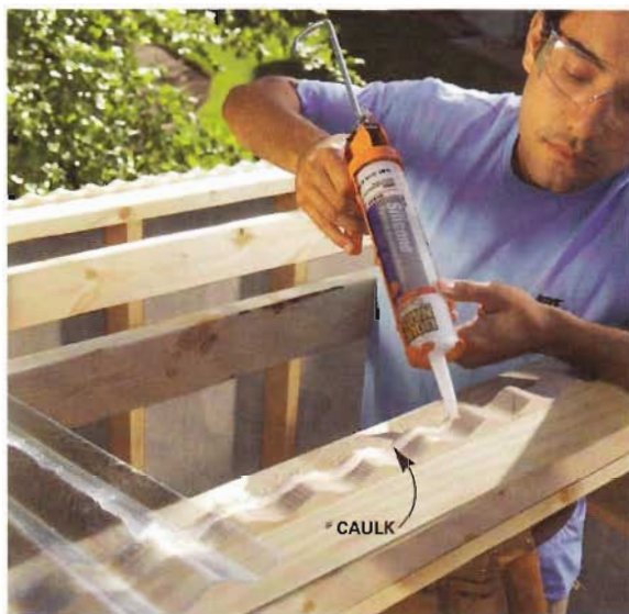
8 Lay a heavy bead of caulk over the plug strip before screwing on the roof panel.
