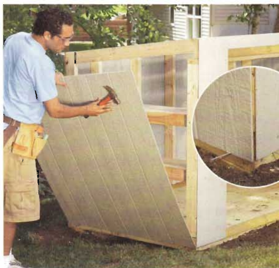
6 Nail on the siding. Support the heavy siding panels with temporary nails placed 1-1/2 in. from the bottom of the floor framing.
