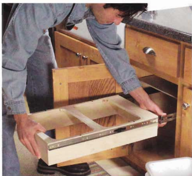
15 Mount the wastebasket carrier and drawer as shown in Photos 10 and 11.
