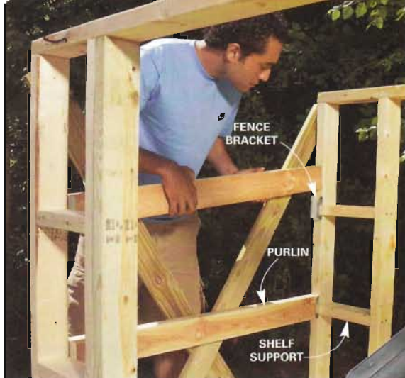
4 Install the purlins. Inexpensive fence brackets make fastening the purlins easy.
